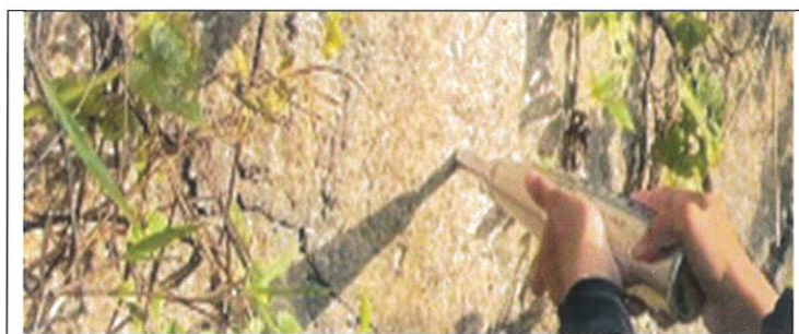
Fig. 3 Collecting rebound data using Schmidt hammer
