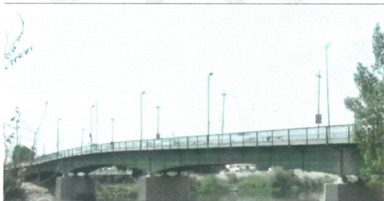
FIGURE 1. A general view of Al Kufa bridge
