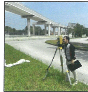
FIGURE 6. Measuring actual data using Total Station
