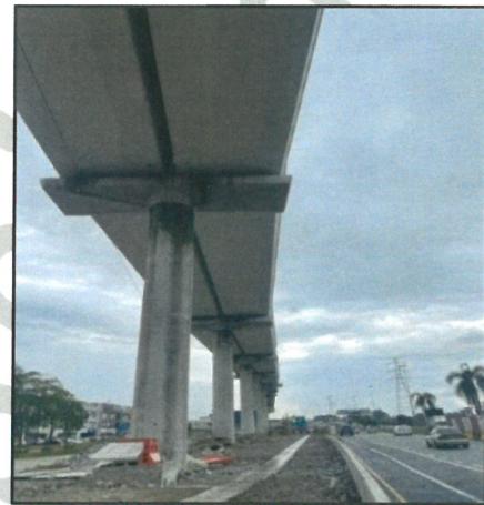
FIGURE 2. Bridge pier structure
