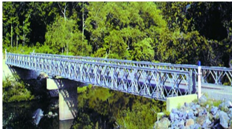
Figure 1.1: Bailey Bridge (Bailey bridge, Inc, 2010)
