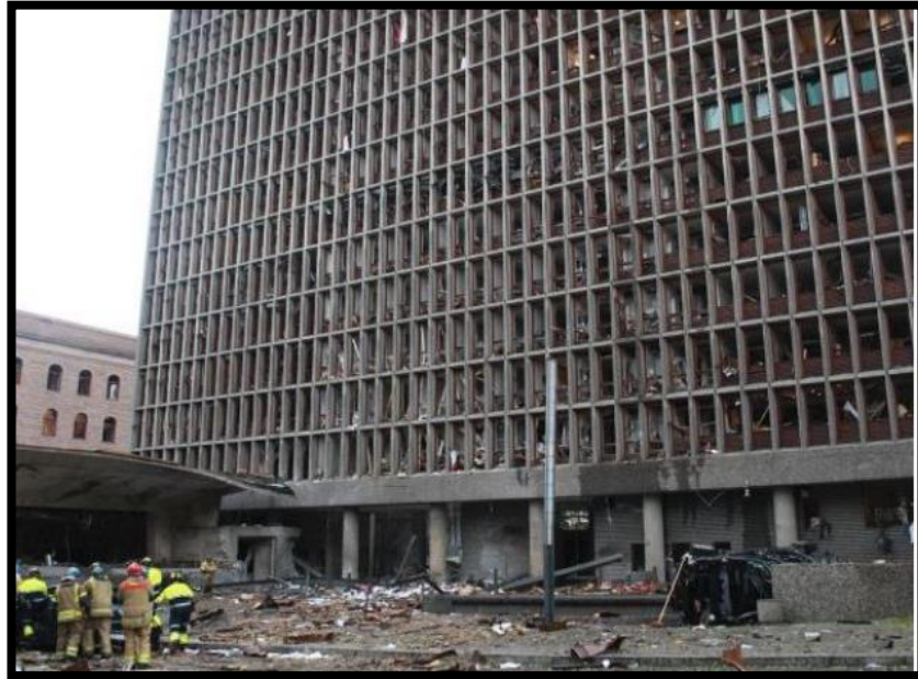
Figure 1.3 Oslo Executive Government Building in Norway attack (Zhang et al., 2017)
